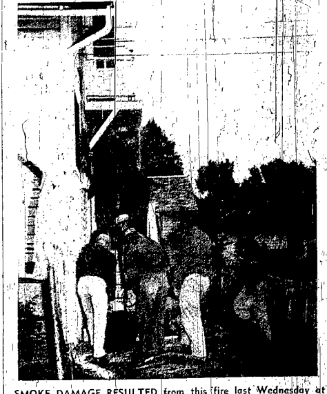
SMOKE DAMAGE RESULTED from this fire last Wednesday at 308 East Ninth when an overheated heating stove in the basement apparently caused a small fire. Wayne firemen quickly brought the blaze under control. The residence is a three-family dwelling owned by Mrs. Izora Laughlin.
